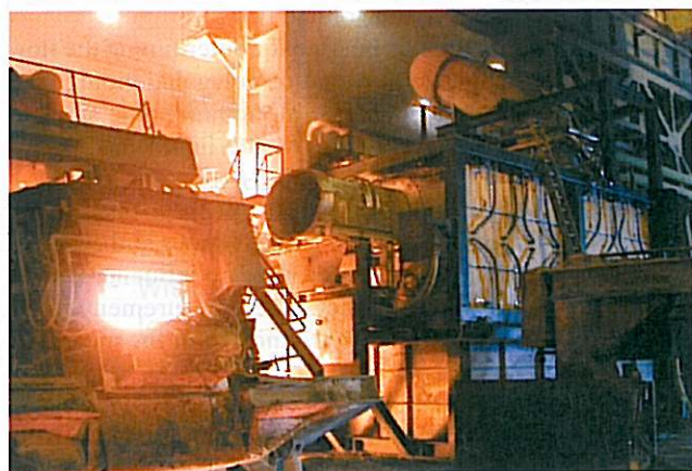
When the EAF roof is swung aside during tapping, the exhaust duct is tilted into the combustion chamber
